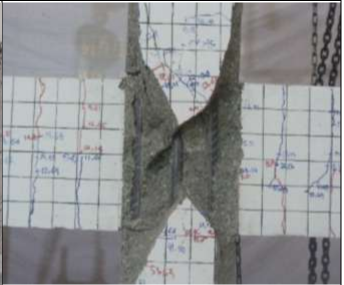
Figure 15. Collapse of Joint BJ-2
